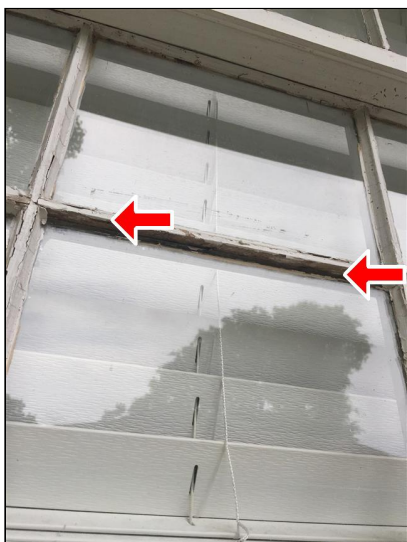
2.2 Item 1(Picture) Missing Window Glazing
