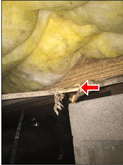
7.2 Item 1(Picture) Frayed Wiring
