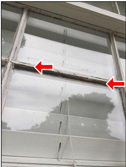
2.2 Item 1(Picture) Missing Window Glazing
