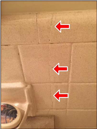
4.1 Item 1(Picture) Cracked Tile
