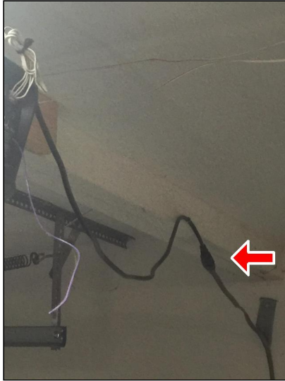
3.5 Item 1(Picture) Garage Door Opener Extension Cord
