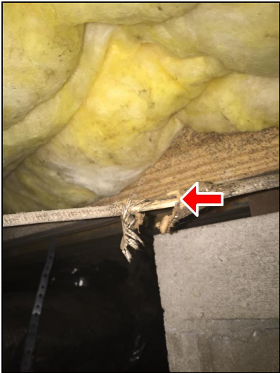
7.2 Item 1(Picture) Frayed Wiring
