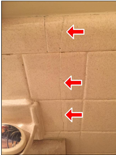
4.1 Item 1(Picture) Cracked Tile
