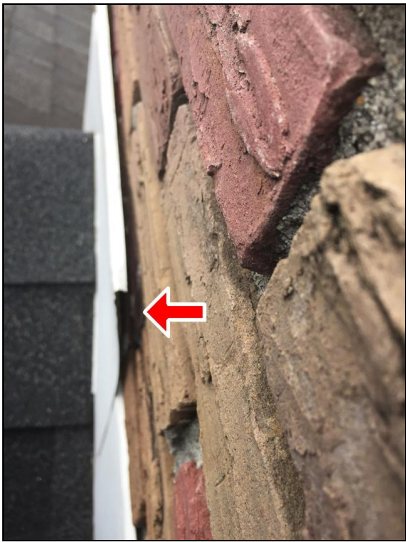
1.1 Item 1(Picture) Loose Chimney Flashing
