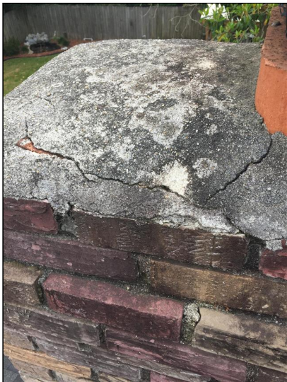
1.2 Item 1(Picture) Cracked Chimney Crown
