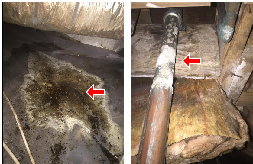
6.0 Item 1(Picture) Standing Water From Waste Pipe Leak 6.0 Item 2(Picture) Leaking Waste Piping
