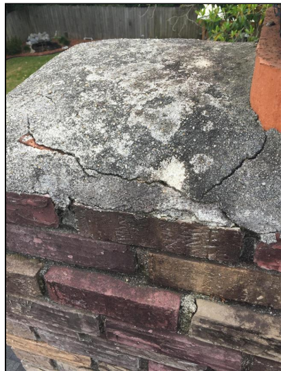
1.2 Item 1(Picture) Cracked Chimney Crown
