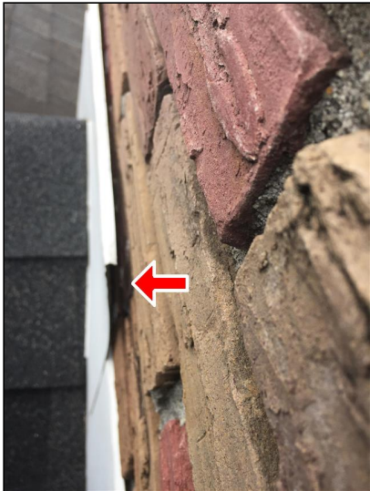
1.1 Item 1(Picture) Loose Chimney Flashing
