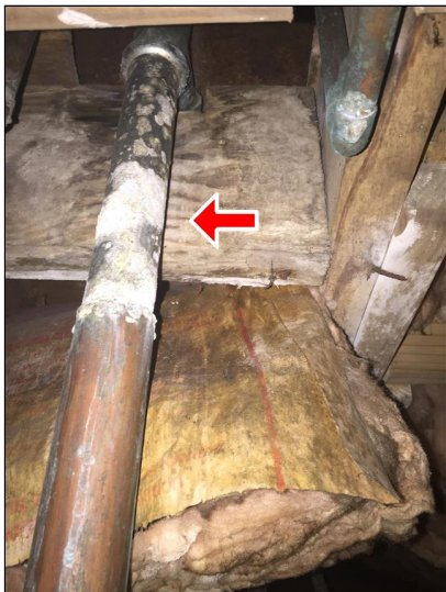
6.0 Item 2(Picture) Leaking Waste Piping
