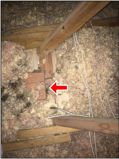
9.0 Item 1(Picture) Missing Insulation
